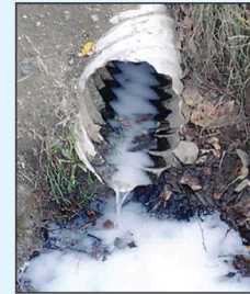
Soap suds exiting a storm sewer pipe.
